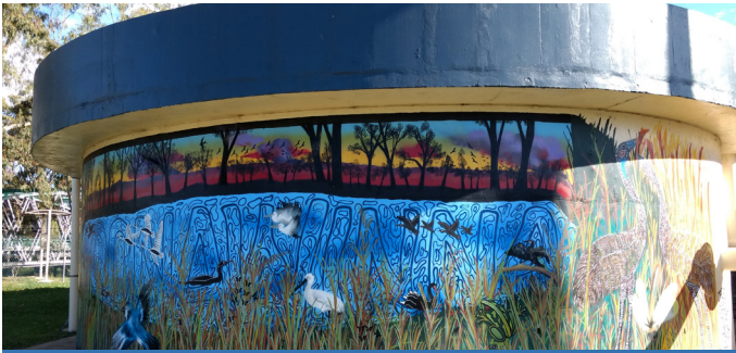
Goondiwindi water reservoir
